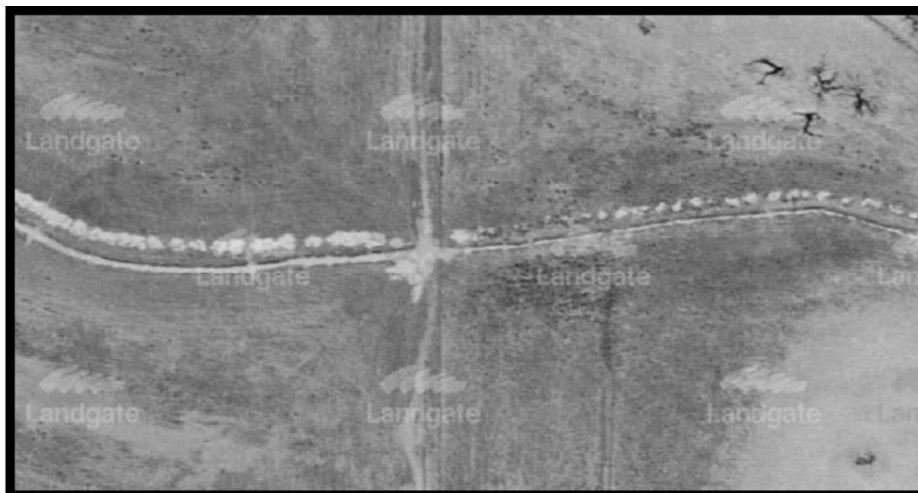
Plate 2: St Leonards Creek Excavation in 1965
